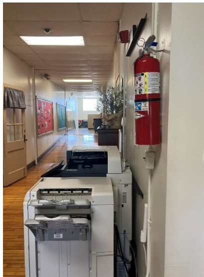
Fire extinguisher mounted too high, obstructed by copier
