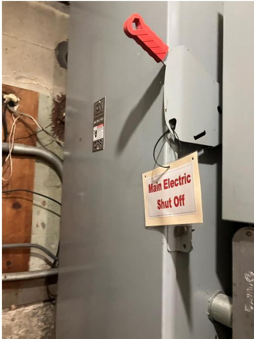
Main shut off switch
