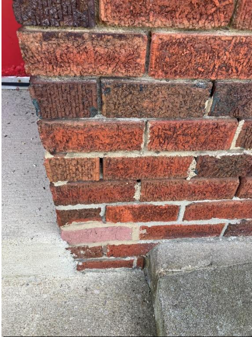
Mortar deterioration
