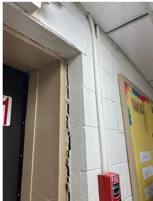
Interior wall cracks
