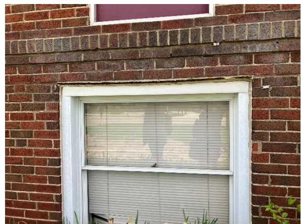
Rusted delaminating lintel
