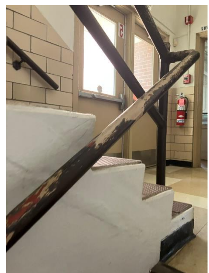
Handrails not compliant with current code
