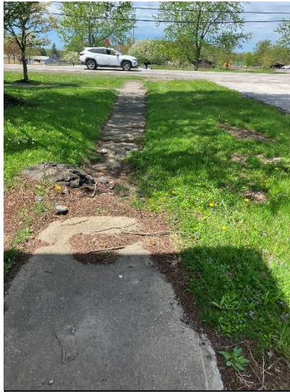
Sidewalk settling
